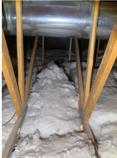
Attic overview (typical insulation)
