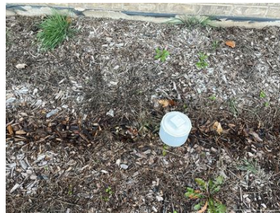
Sewer Cleanout (Exterior)
