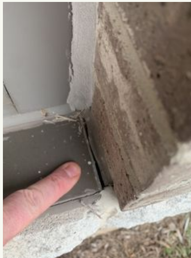
typical failed sealant at many areas
