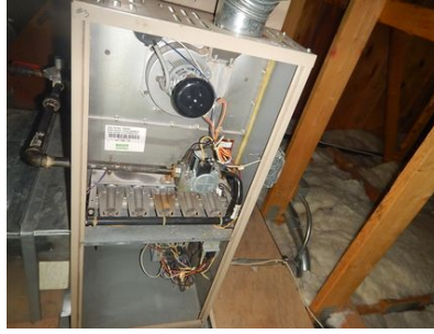
Furnace with cover removed
