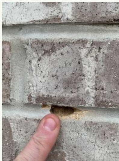
rear of building
