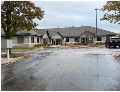
Front view of building
