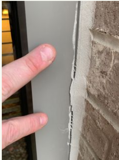
typical failed sealant at many areas
